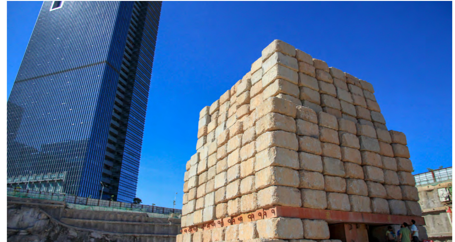
Static Load Testing Site in CTC Xiamen Hongye Co., Ltd.
