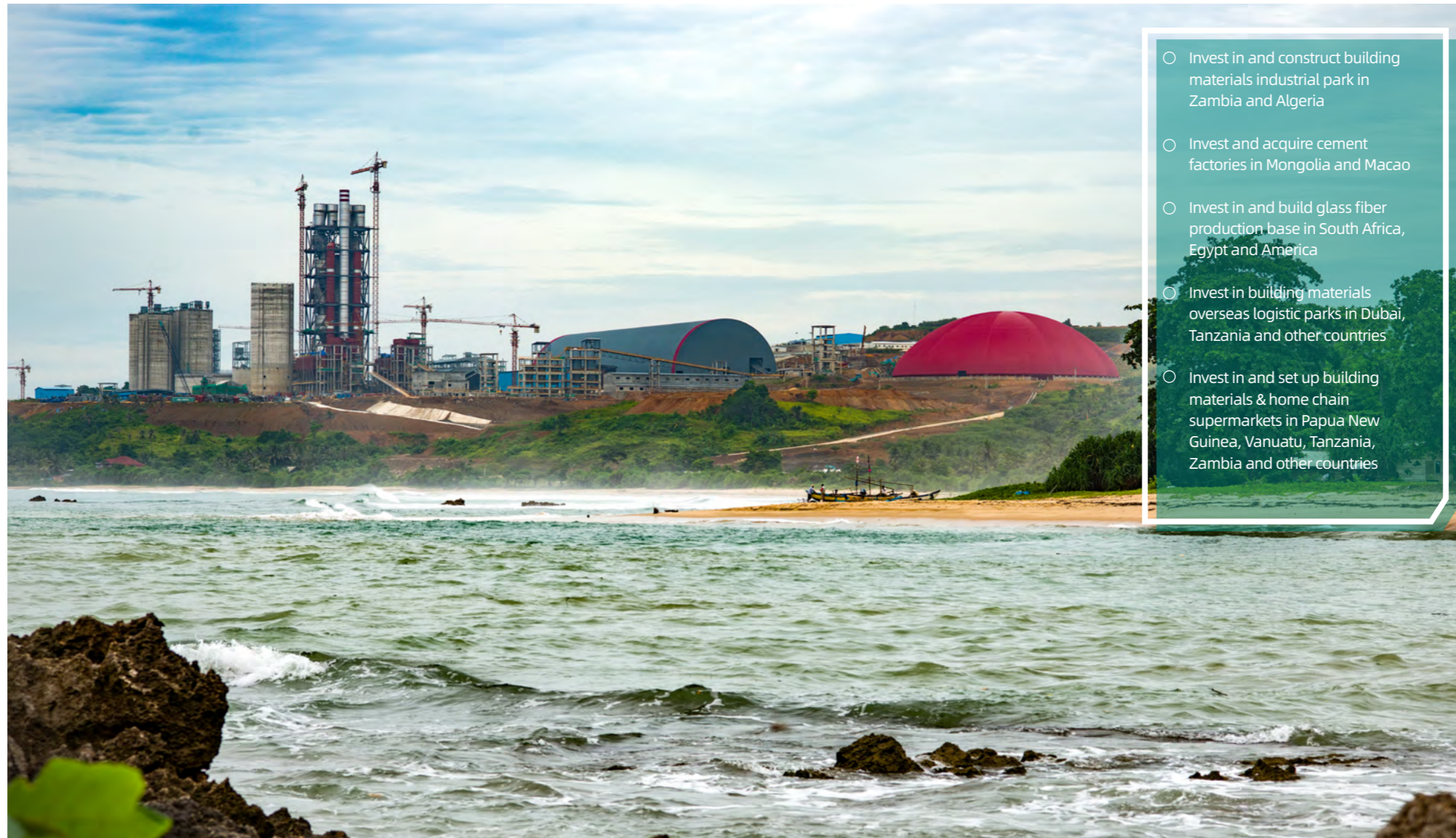
Indonesia Baya 10,000TPD cement production line undertaken by Sinoma International Engineering Co., Ltd.
