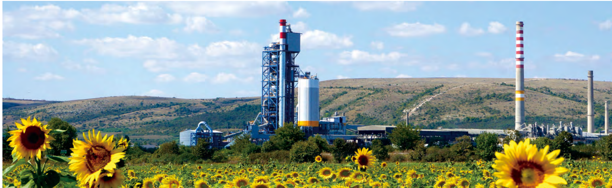
☉ Panorama of Bulgaria Devnya Project
